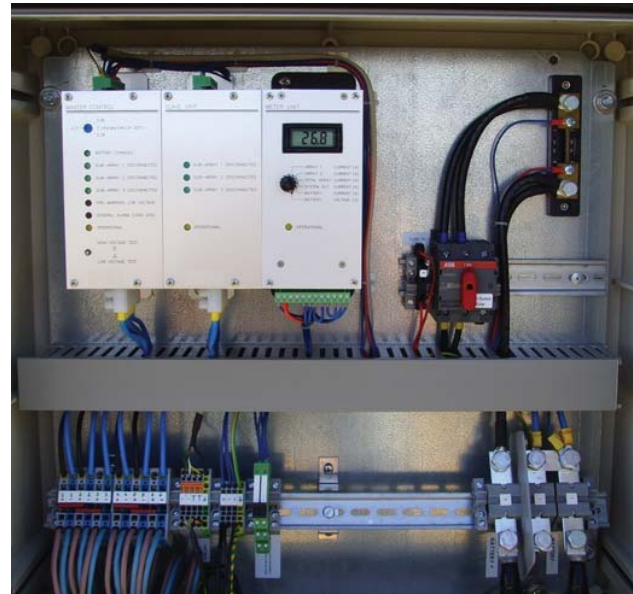
Figure of a typical enclosure with 1 master control, 1 slave unit and 1-meter unit
