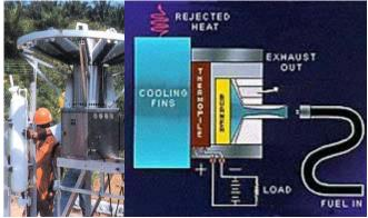
Natural gas pipelines are often protected with current supplied from thermoelectrically generators fuelled with natural gas tapped from the pipeline via suitable pressure reducing and valve arrangements.
